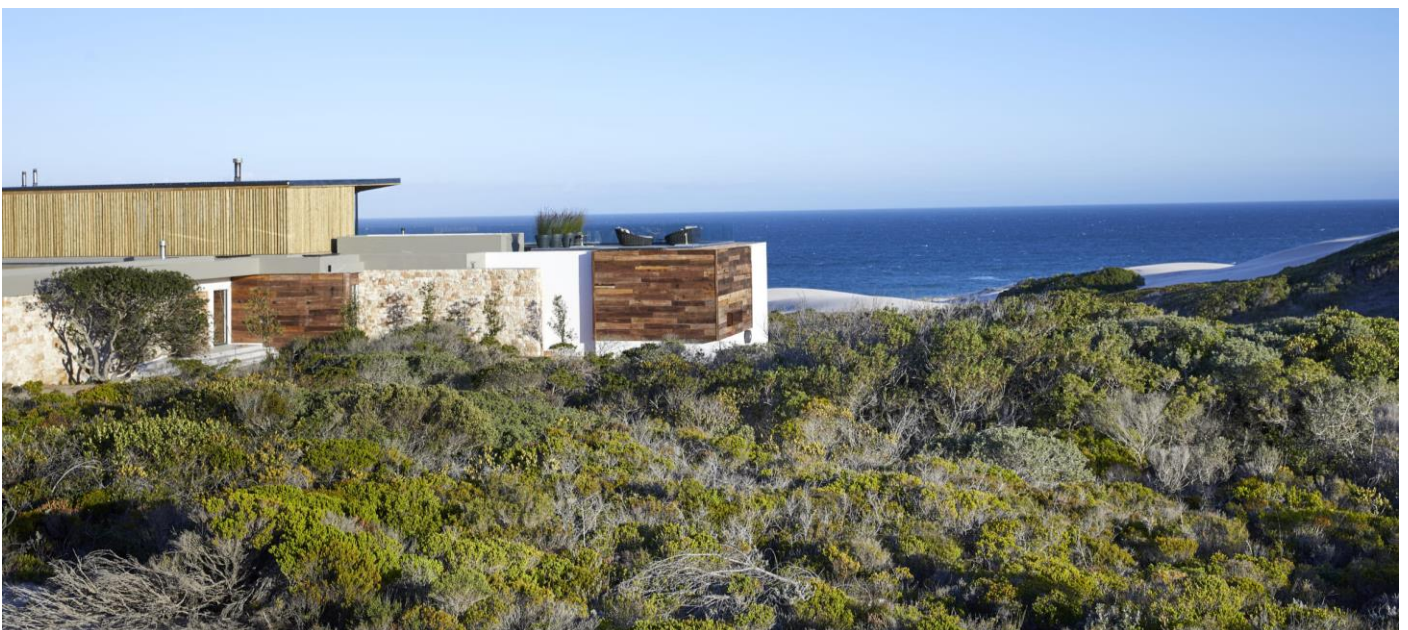
Morukuru Beach Lodge site and view
